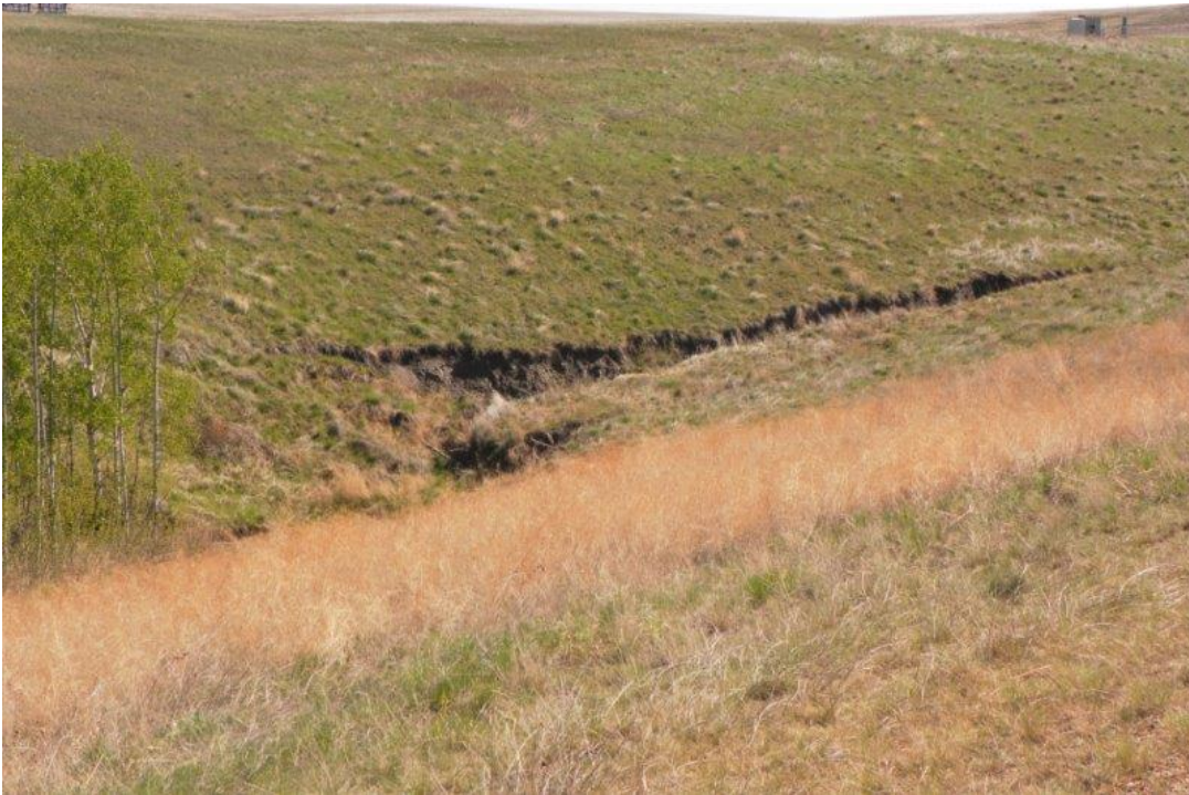
Clark Coulee still a washout and extensive backsloping
